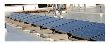
For Baker Labs on the SUNY Environmental Science and Forestry campus, we installed a 23 KW PV array as part of the architectural design of the building. Mounting the solar panels to engineered steel beams on the building's exterior provided optimal performance of the solar modules and shade for the windows in summer. The building now produces 20% of its power by renewable sources.
